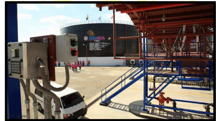
Storage complex in Corinto
